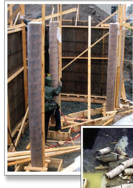
Cardboard columns, even when wrapped in poly, fail in moisture and rain
