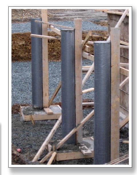
Fast-Tube<sup>™</sup> is manufactured from high strength polyethylene, and is undamaged by moisture.
