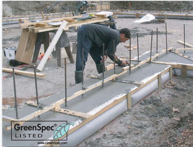
Fastfoot®, the patented footing form and stay-in-place membrane prevents rising damp & improves indoor air quality.
