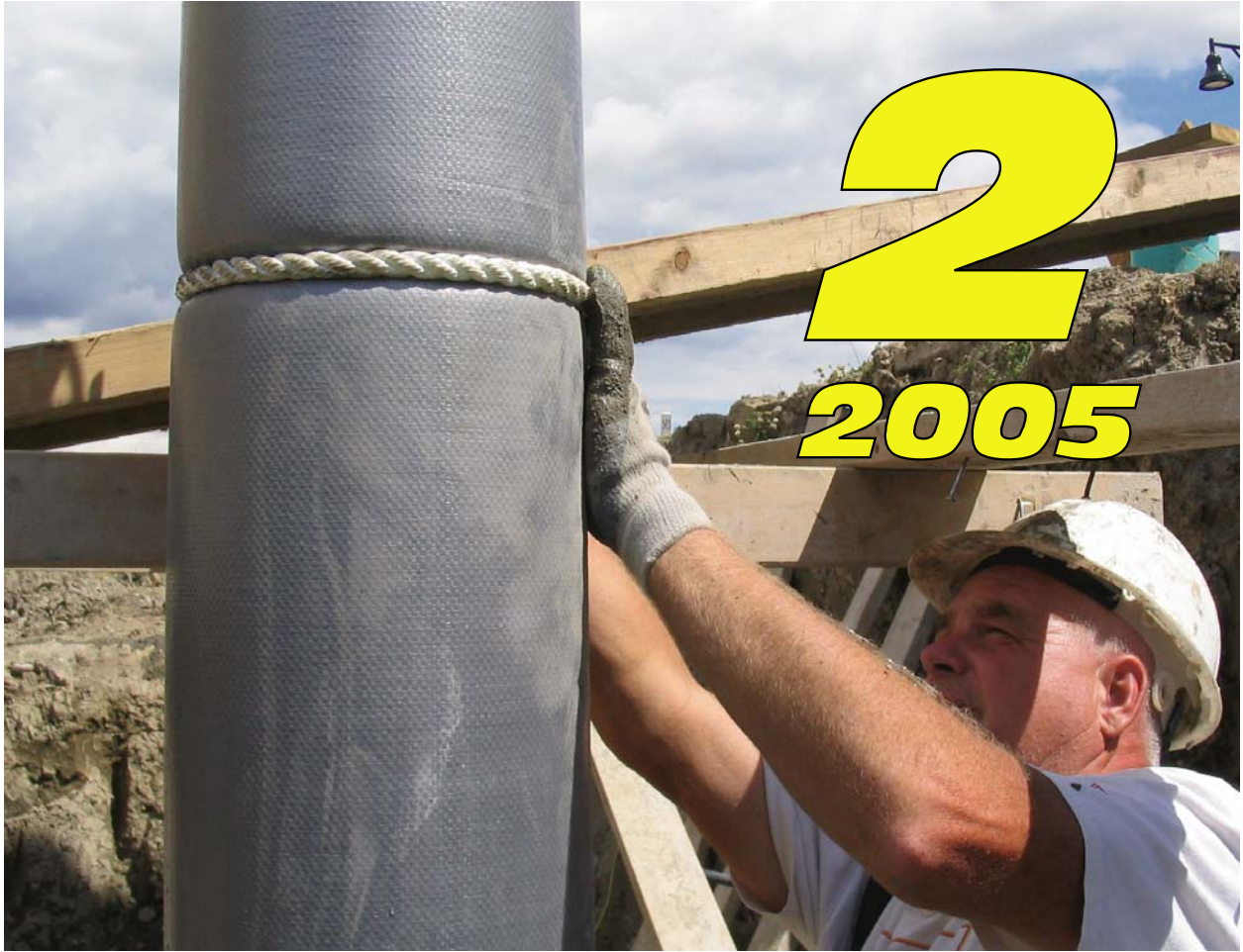
Ron Kautzma, Sunset Builders, produces decorative columns with Fast-Tube™.
