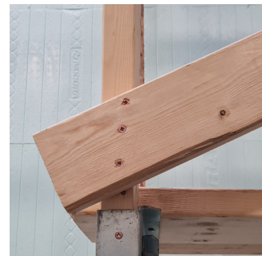
Figure 12: Connection of diagonal brace at end post.
