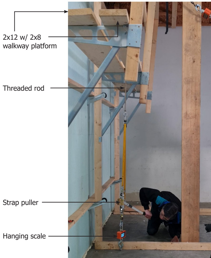
Figure 7: Application of vertical load test
