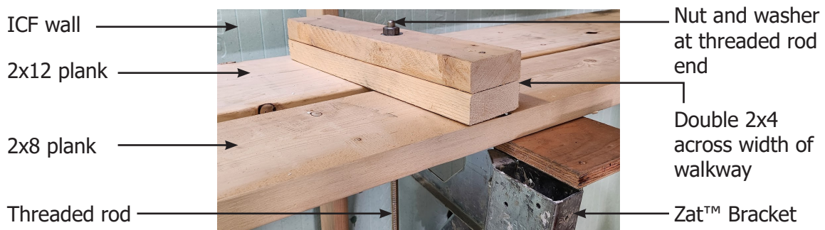
Figure 8: View of threaded rod connection to walkway platform.
