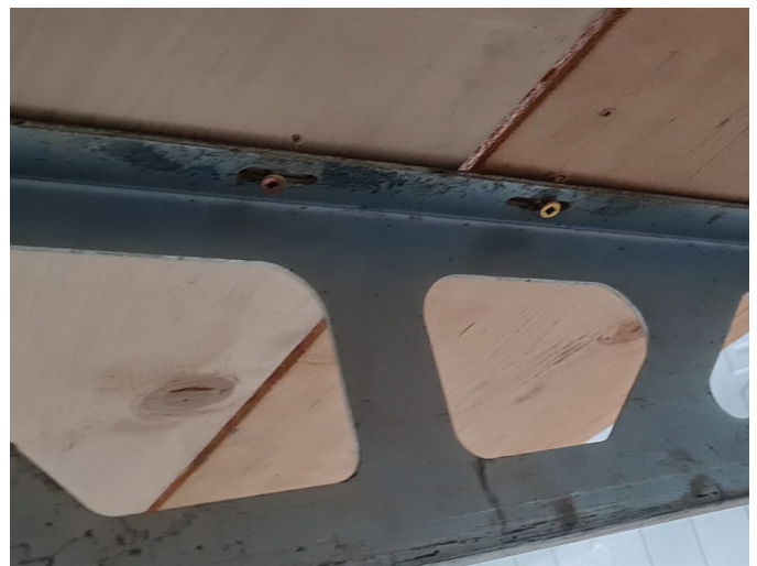
Figure 5: Zat™ Bracket connection to walkway platform
