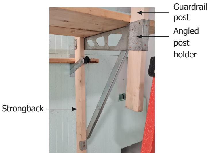
Figure 4: Zat™ Bracket connection to Strongback and guardrail
